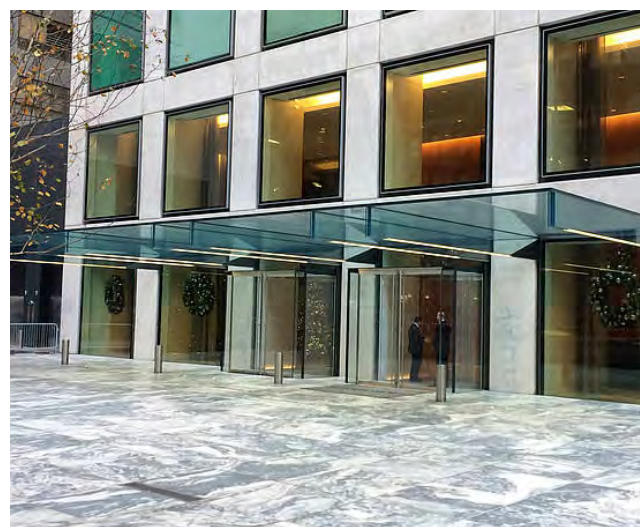
5. DROP-OFF CANOPY CLEAR STRUCTURAL GLASS
